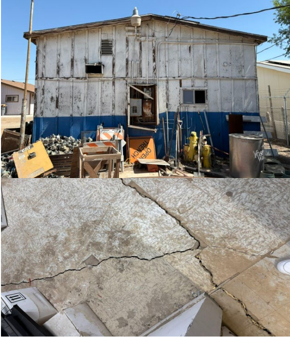
Shop & Storage Building Repairs
